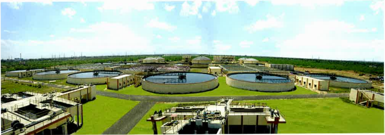
180 MLD STP, Pirana, Municipal Corporation, Ahmedabad India's First Largest STP with Diffused Aeration and PLC - SCADA System
