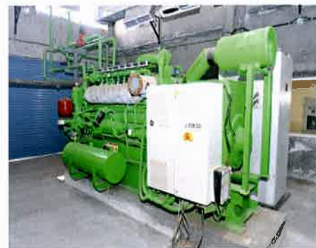
600 KWe Capacity Bio Gas Power Plant at 84 MLD STP, Variav for SMC, Surat
