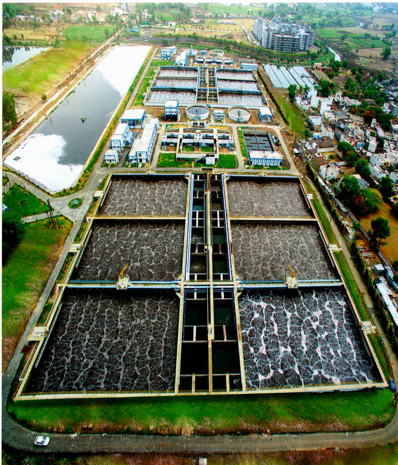
245 MLD STP for Indore Municipal Corporation, World's first Largest Single Stage Biological SBR Based STP
