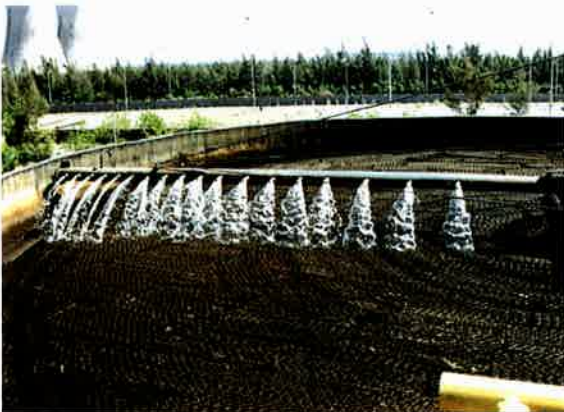
Bio-Tower Installation for Effluent Treatment Plant, RELIANCE, Hazira
