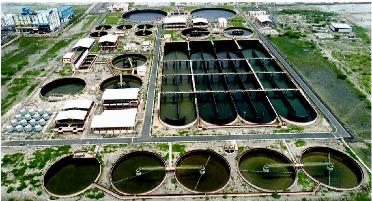
40 MLD CETP at Dahej for Gujarat Industrial Development Corporation
