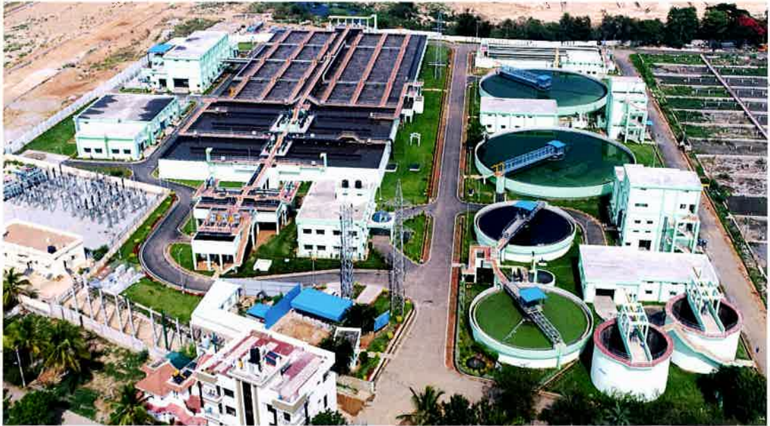
40 MLD Capacity STP based on BNR System at Raja Canal for Bangalore Water Supply and Sewerage Board
