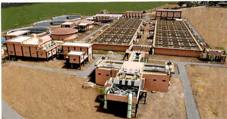
84 MLD Two Stage Biological (UASB + MBBR) STP at Variav for Surat Municipal Corporation
